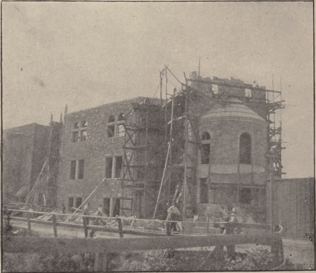
ALMOST READY FOR THE ROOF.
